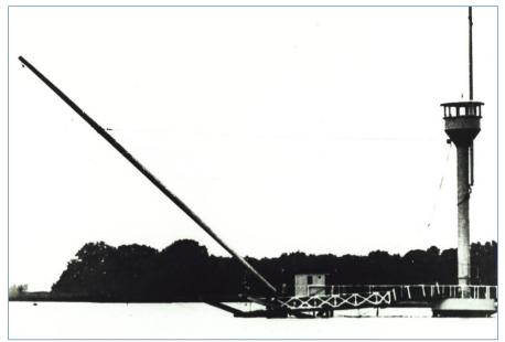
Figure 6: Mast with additional enclosure added to the upper level after its original placing (IMU)
